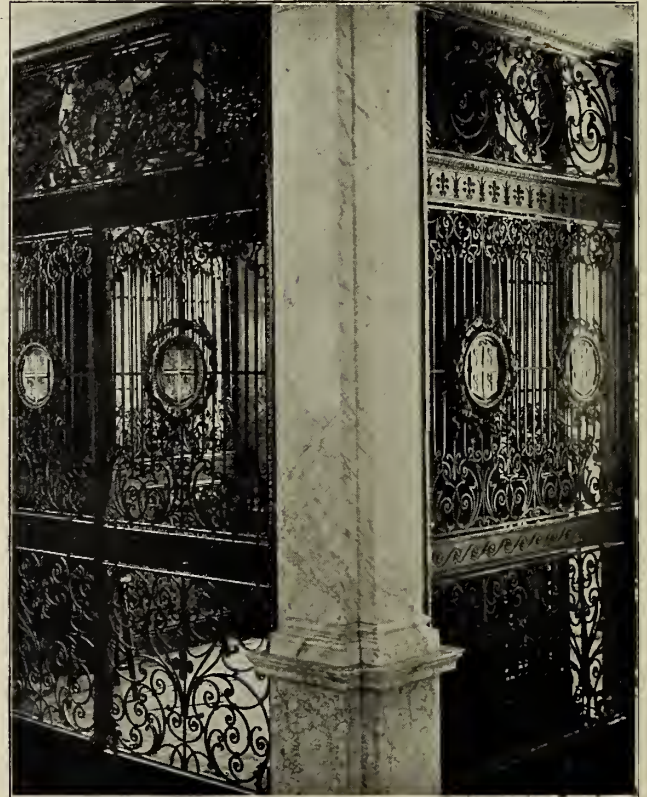
C.—ELEVATOR INCLOSURES, OLD COLONY BUILDING, CHICAGO. Wrought Iron, Hammered Leaf.
